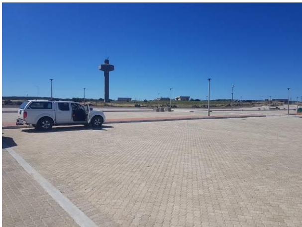
Image 4: Completed car park area.
