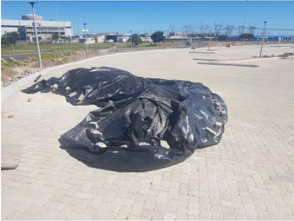
Image 9: Material stockpile protected from wind and water erosion.
