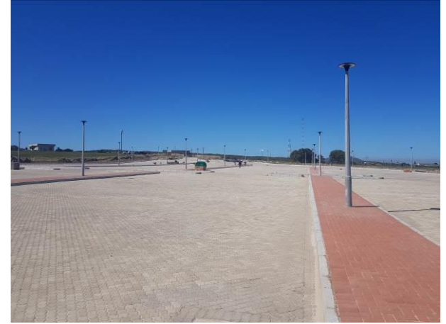
Image 3: Completed car park area with, lamps installed.
