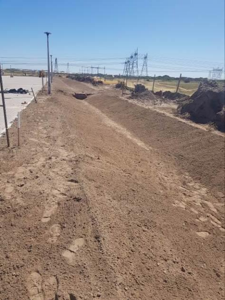
Image 10: Construction of the V-drain.
